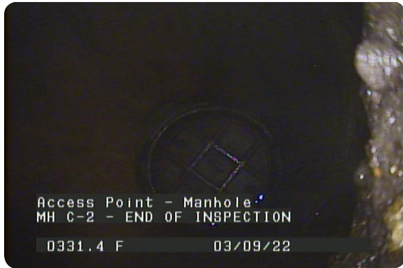
Access Point - Manhole at 331.4 feet | MH C-2 - END OF INSPECTION
