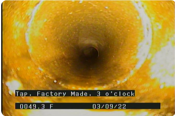
Tap, Factory Made at 049.3 feet, 3 o'clock, 4 in
