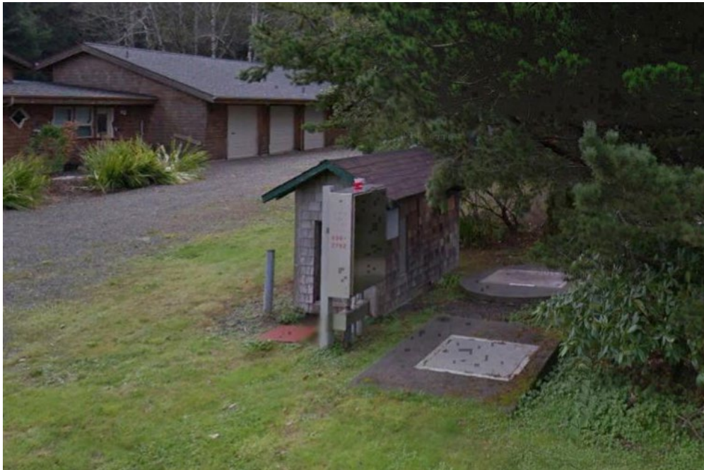
Webb Avenue Pump Station
