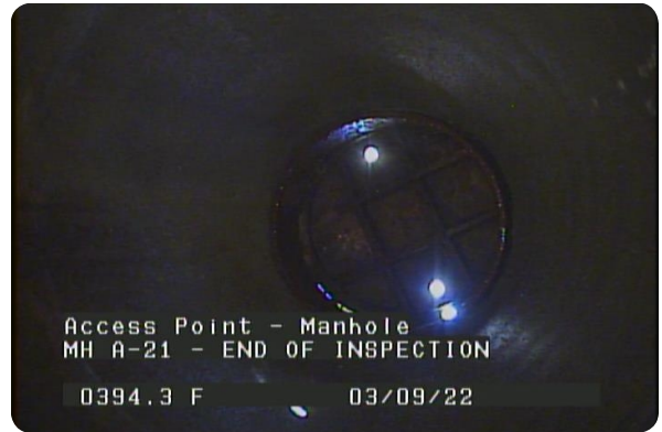
Access Point - Manhole at 394.3 feet | MH A-21 - END OF INSPECTION
