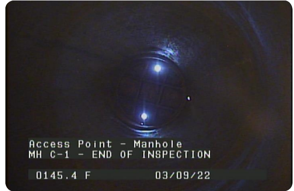
Access Point - Manhole at 145.4 feet | MH C-1 - END OF INSPECTION
