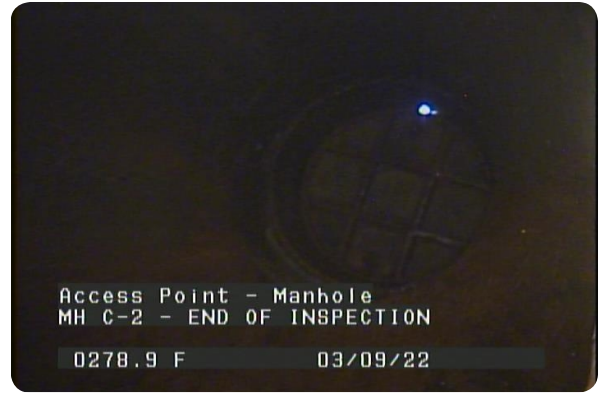
Access Point - Manhole at 278.9 feet | MH C-2 - END OF INSPECTION
