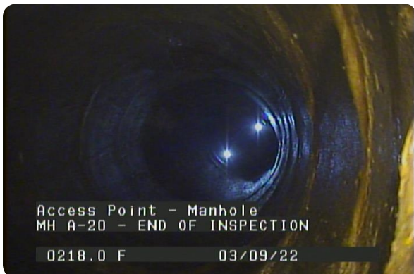
Access Point - Manhole at 218.0 feet | MH A-20 - END OF INSPECTION
