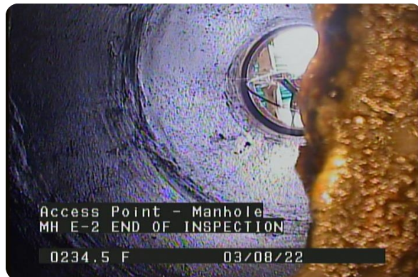
Access Point - Manhole at 234.5 feet | MH E-2 END OF INSPECTION
