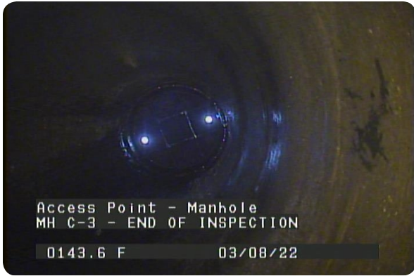
Access Point - Manhole at 143.6 feet | MH C-3 - END OF INSPECTION
