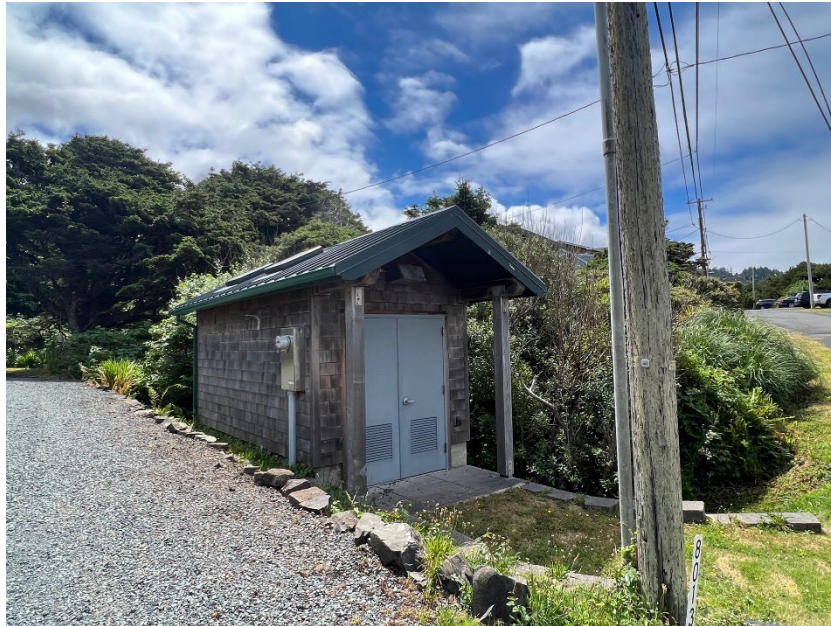
Sally's Alley Pump Station Control building
