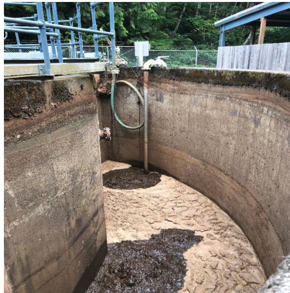
Aerobic Digester No. 2
