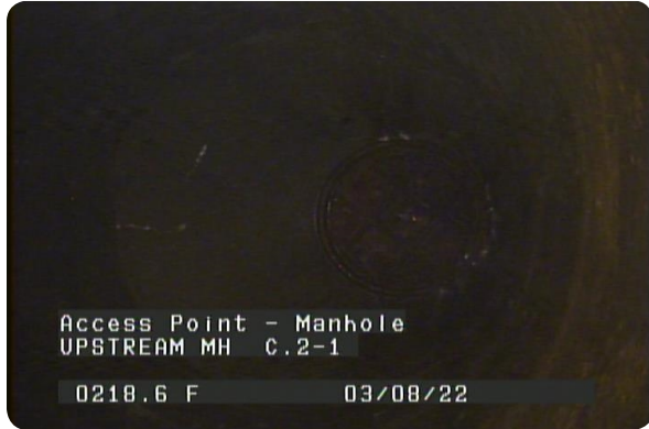
Access Point - Manhole at 218.6 feet | UPSTREAM MH C.2-
