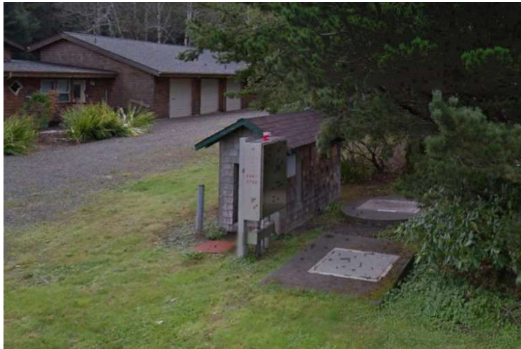
Webb Avenue Pump Station
