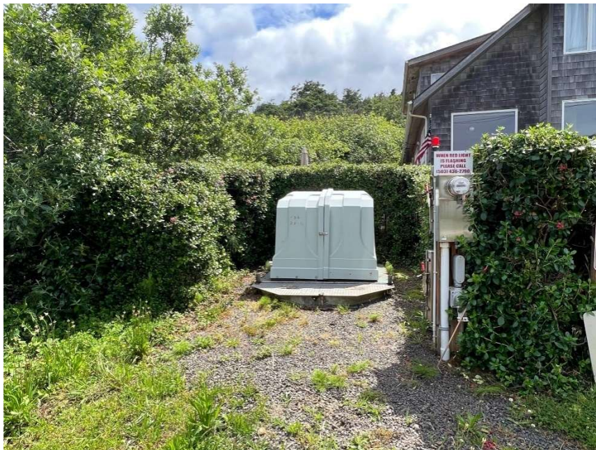
Asbury Pump Station
