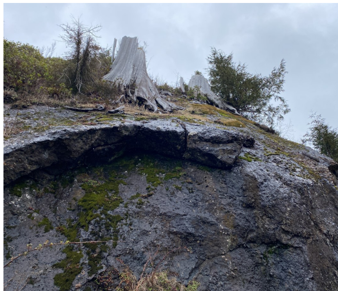
Rock wall along Shingle Mill XO road (photo credit: NCLC)
